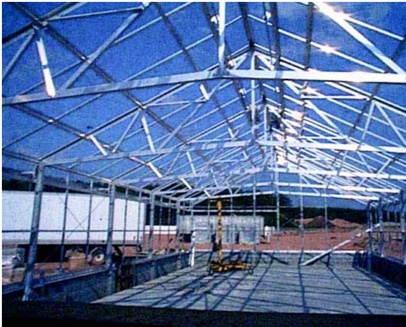
FIG 15. Aluminum-framing under construction
