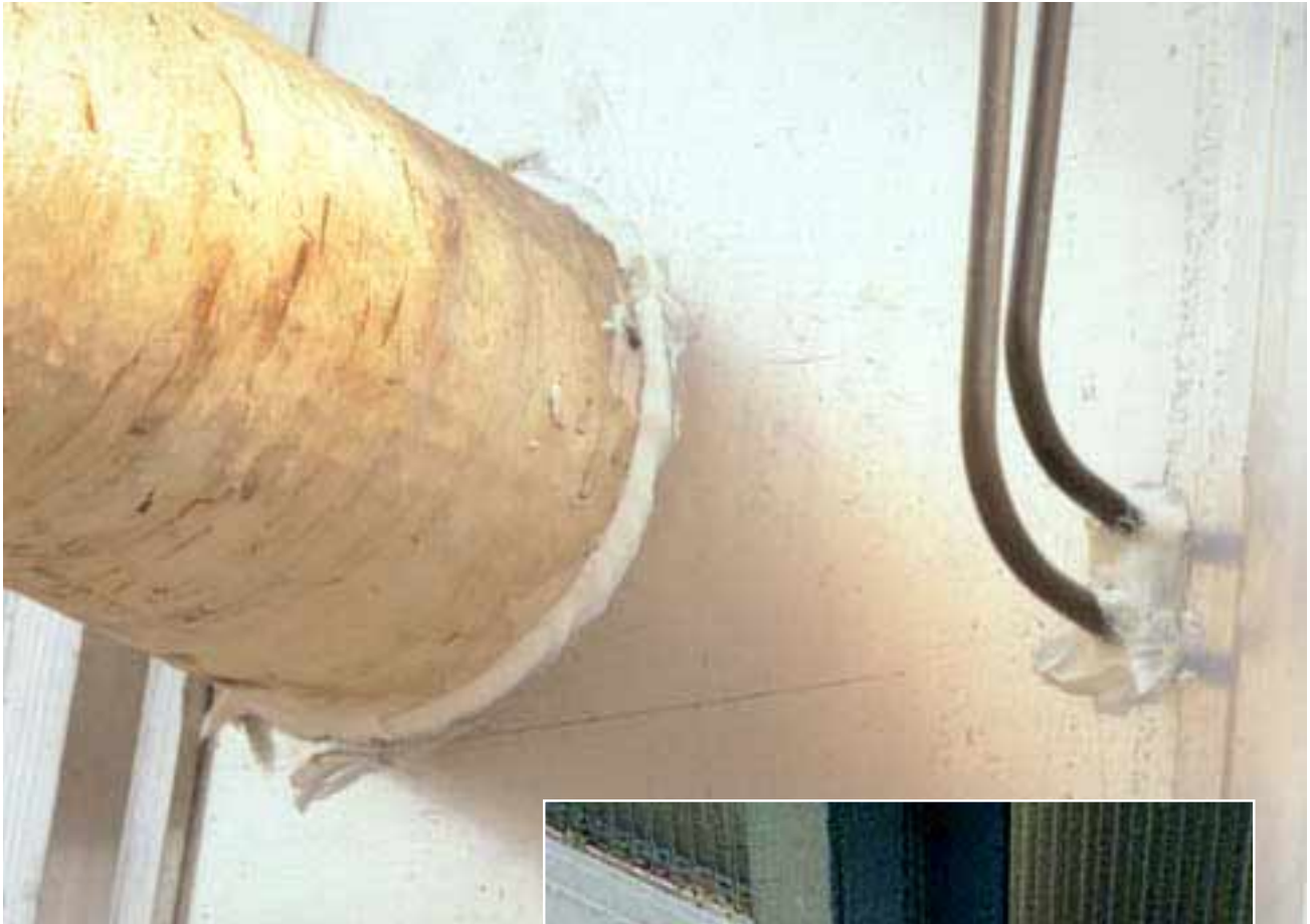
FIG 1. Caulking around service intrusions
