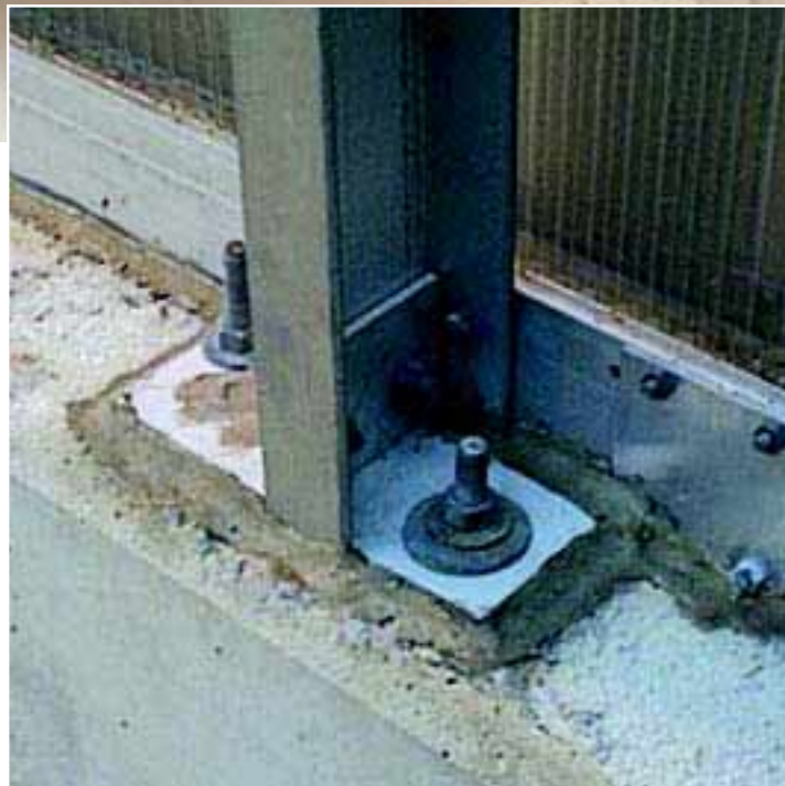
FIG 2. Sill caulking
